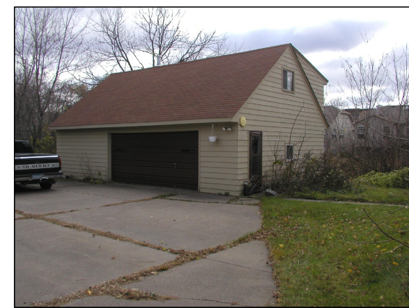
GARAGE AT 3253 OLD HIGHWAY 8
